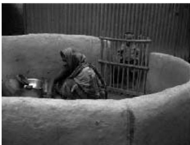
**Figure 8 Mud barrier around a cooker**
