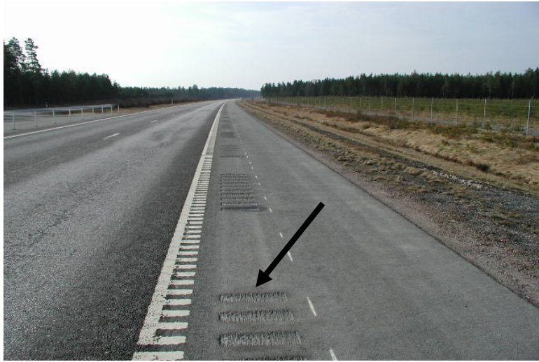
Figure 3 Rumble strip milled into the road surface at the shoulder.
