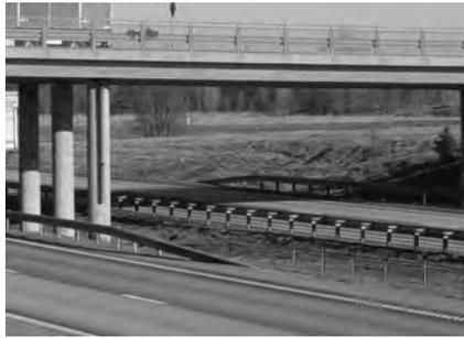
**Figure 2.** Bridge pier with W-beam guardrail and cable guardrail.
