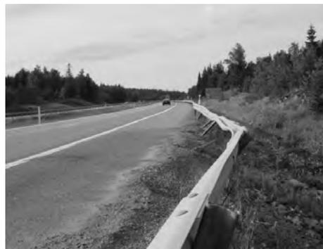
**Figure 1.** 5 star vehicle override a W-beam guardrail.
